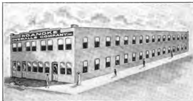
VIEW OF THE PLANT
