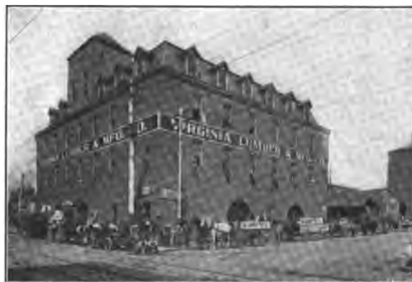
PARTIAL VIEW OF PLANT
