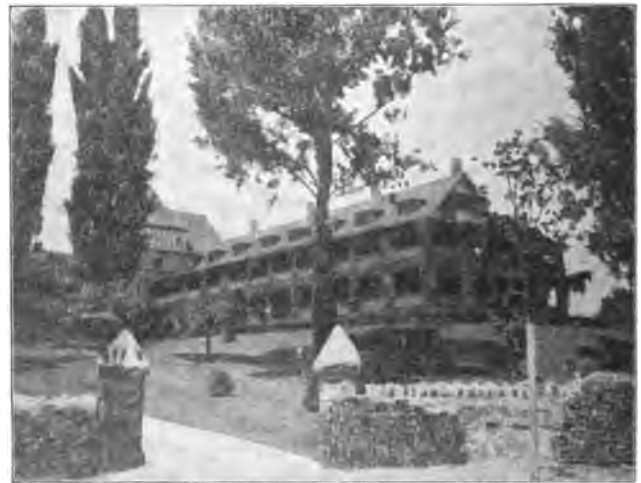
ENTRANCE FROM NORFOLK &amp; WESTERN STATION
