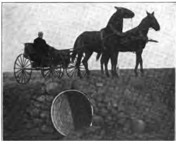
A HIGHWAY CULVERT
