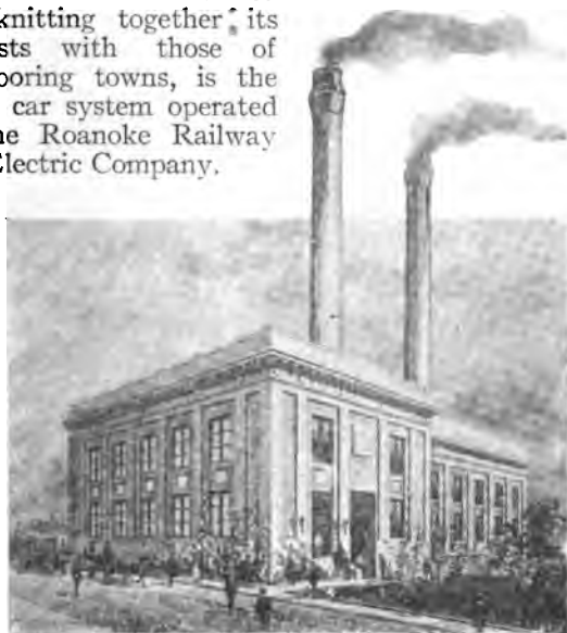
STEAM POWER PLANT
