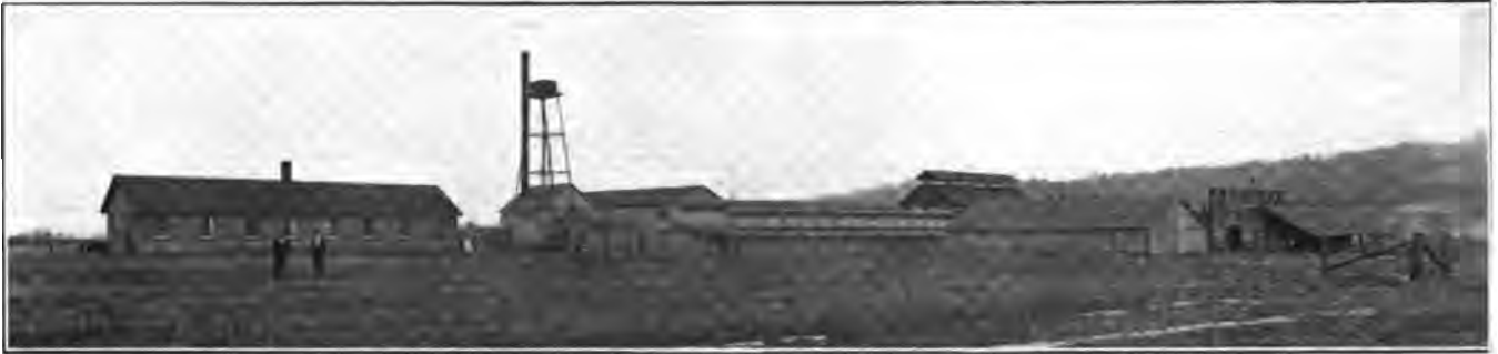
VIEW OF PIERPONT BRICK WORKS FROM MACADAM ROAD, LOOKING EAST
