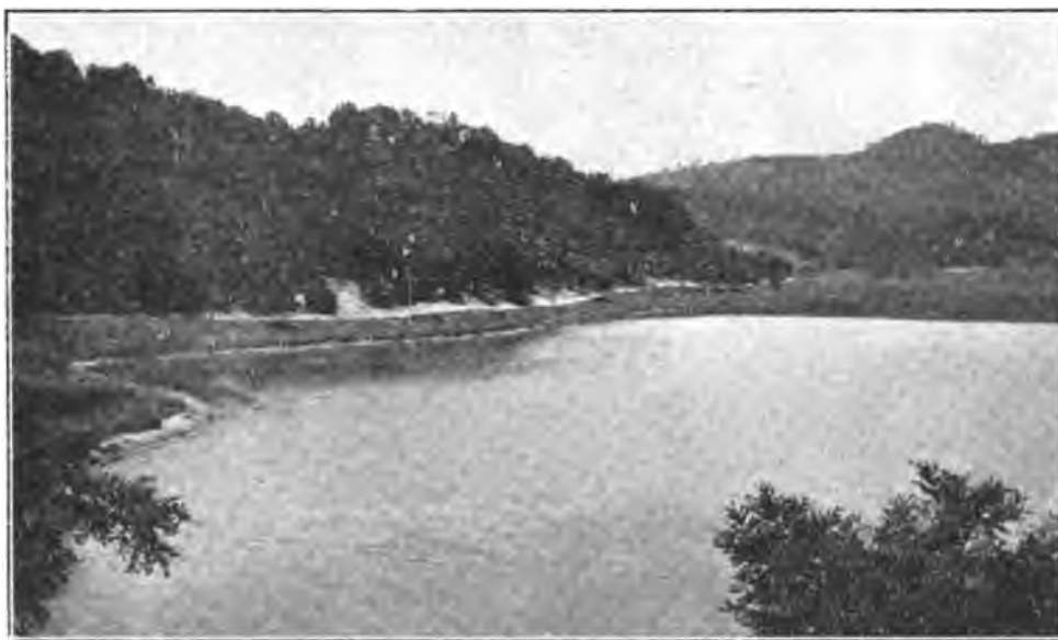
RESERVOIR OF VINTON-ROANOKE WATER COMPANY 120,000,000 Gallons Capacity
