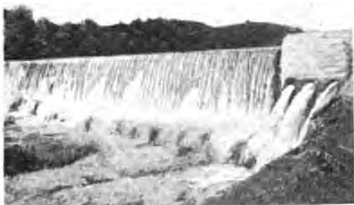
WATER POWER PLANT
