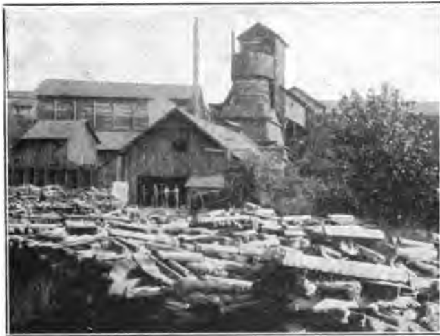
COLD BLAST CHARCOAL FURNACE, FOSTER FALLS, VIRGINIA (Type of Furnace Existing Before the War)
