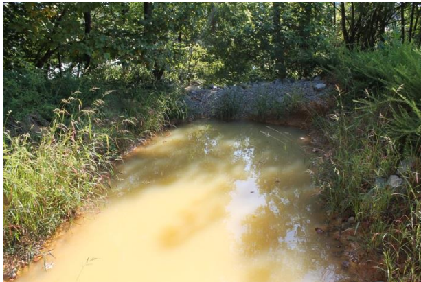
Storage Yard Sediment Trap
