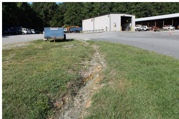
Eroded Stormwater Conveyance Channel
