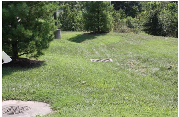
Stormwater Drain Inlet on South End of Fleet Services Center
