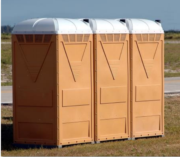
These portable toilets are appropriately placed on level ground in a grassy area, well away from any components of a storm drainage system. Anchoring to prevent tipping is encouraged.
