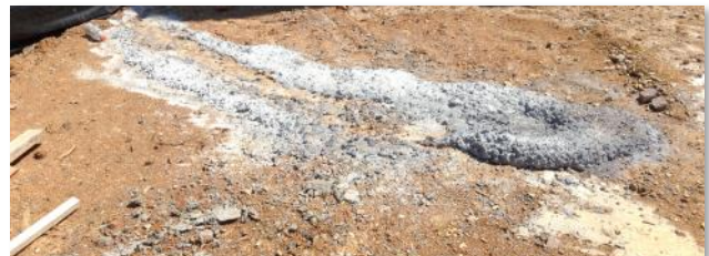
Concrete has been inappropriately washed out directly onto the ground, which is another type of illicit discharge.
