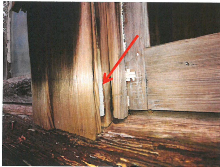
The Felt Paper located under wooden shingle siding on the shed behind the home was found to be Asbestos Containing by the laboratory.
