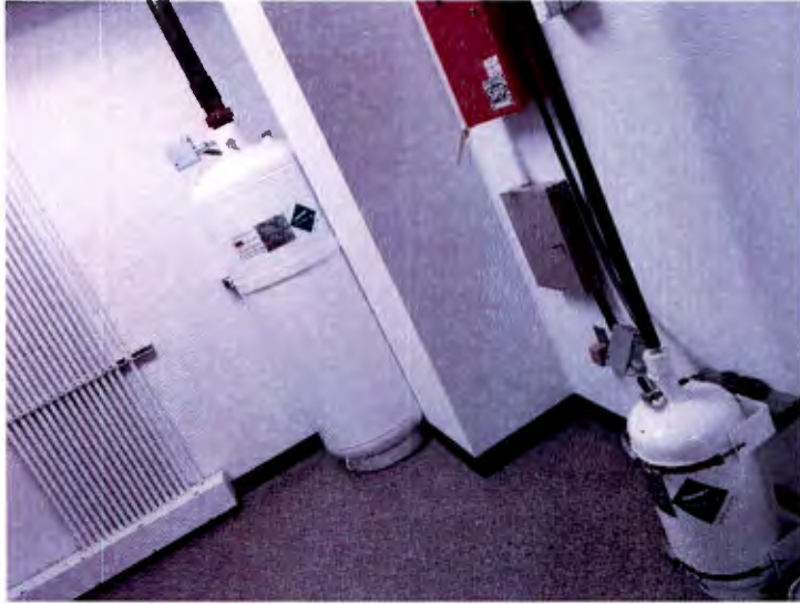
Electrical Room- 5925 Cove Road Roanoke, Va
