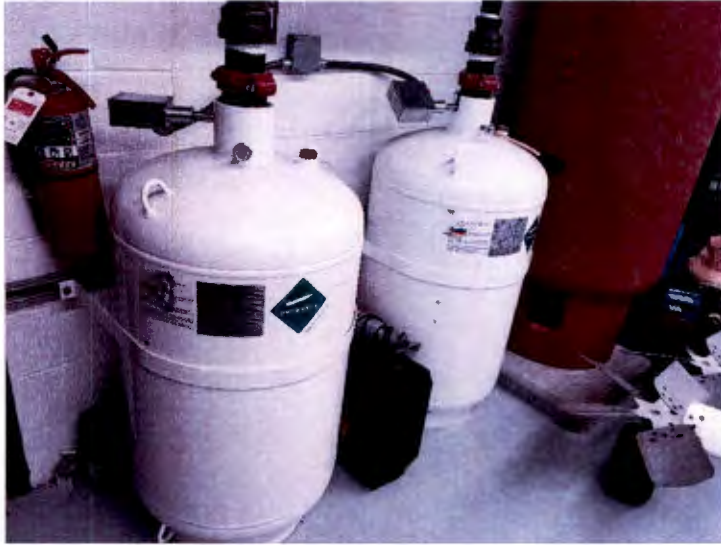
Water Pump Room-5925 Cove Road Roanoke VA
