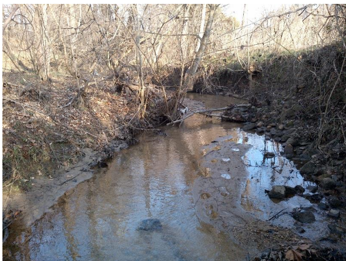
Photo 10. "Very High" erosion along the left bank and "High" erosion around Station 25+00 (looking downstream). Grade back both banks and install rock toe along the right bank. Use local material when possible (see Sheet 3 of Conceptual Drawings).
