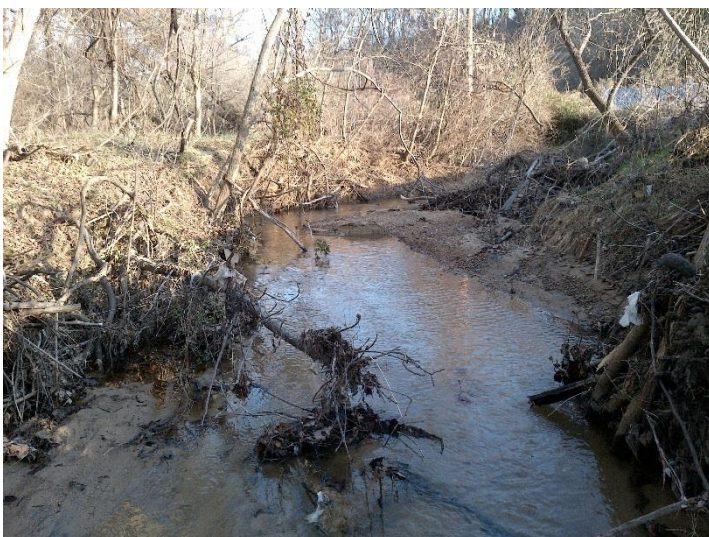
Photo 9. "Extreme" right bank at approximately Station 24+00. Install toe wood for slope stabilization along right bank. Grade back bank on left (see Sheet 3 of Conceptual Drawings).
