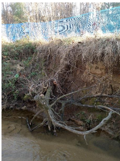
Photo 8. "High" erosion along the left bank close to the Wolf Creek Greenway around Station 23+50. Grade back bank and install bankfull bench. Install rock toe along bank in the bend to provide slope stabilization (see Sheet 3 of Conceptual Drawings).
