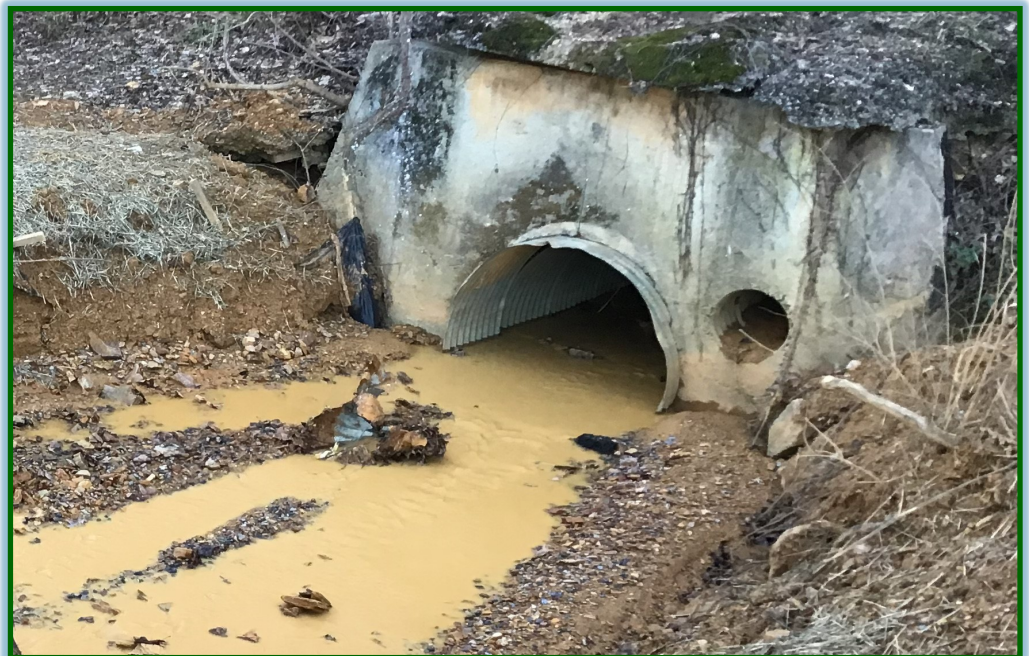
Stream impacts usually result when sediment-laden stormwater runoff leaves an active construction site
