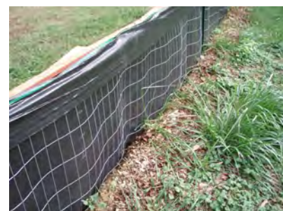
Silt fence is often used as perimeter control
