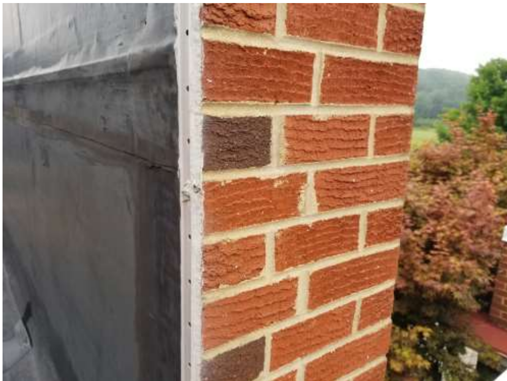
Photograph #0004 EPDM Portion—Grey caulk (5% Chrysotile) at termination bar
