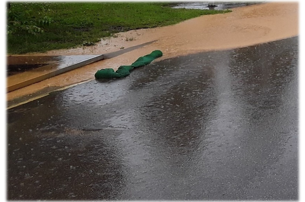
Unchecked sediment leaving a construction site indicates that erosion and sediment controls are either absent or improperly installed or maintained. This is unfortunate, because the sediment will end up in the nearest waterway, and all of the County’s waterways are already impaired due to sediment pollution.
