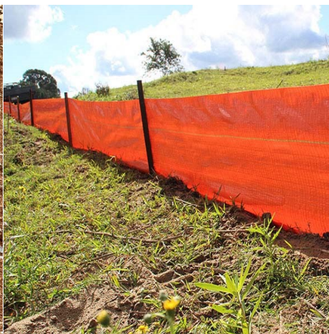
Entrench silt fence into the ground to prevent sediment from escaping beneath it; this keeps your dirt on your site.
