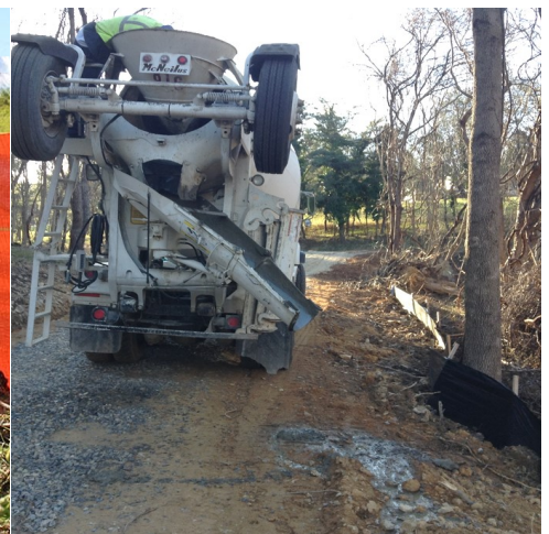
Use a concrete washout! Make sure that it is accessible, and replace it when it gets full.
