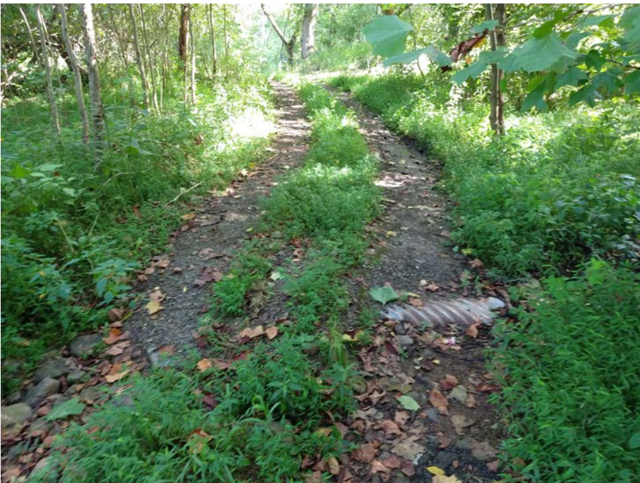
Picture 6 – Note exposed steel culvert
