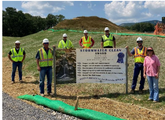
Appalachian Power's Glenmary Substation project wins the Roanoke County Stormwater Clean Award for its proactive efforts regarding erosion and sediment control.
