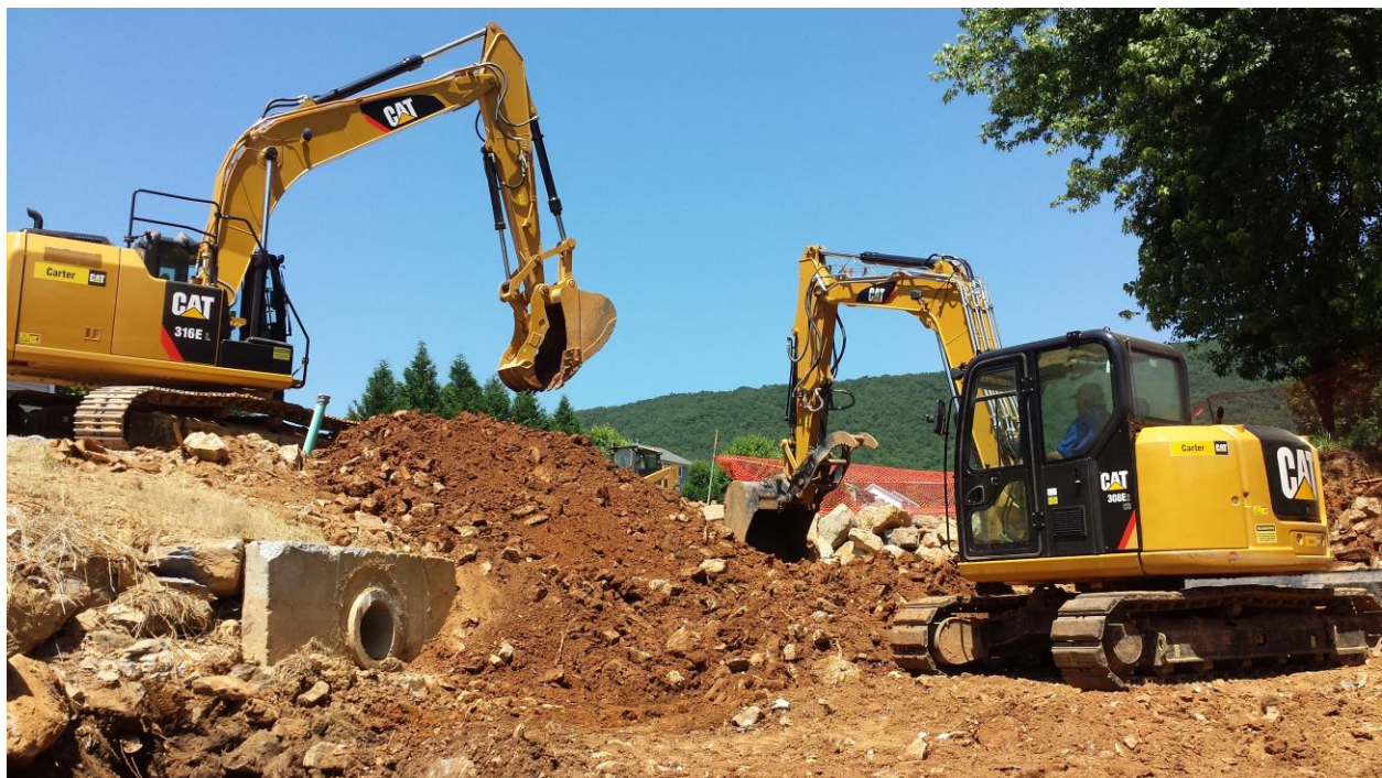
County drainage crew improving an existing storm drainage system.
