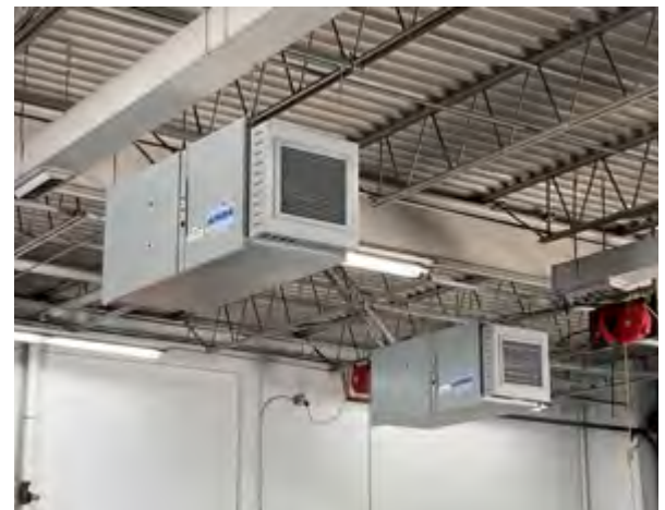
Above: New air filtration units at most Fire and Rescue stations filter cancer-causing fumes and contaminants to help keep staff and volunteers healthy.
