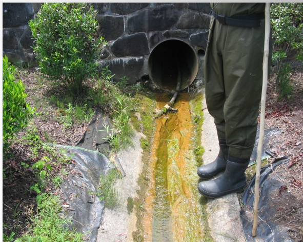
Storm drainage pipes often discharge pollutants, such as bacteria, grease, sediment, and household chemicals into local waterways.
