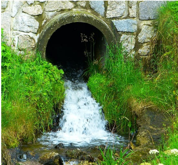
Pollutants from restaurants often enter local streams by way of the storm drainage system, which includes inlets, pipes, ditches, and roadway gutters.
