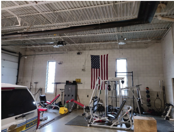
Figure 7, showing the joists sloping from plan south to plan north (Left to right).
