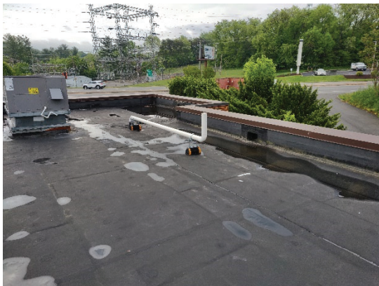
Figure 20, showing one of the roof drains and scuppers. With the slope of the roof.
