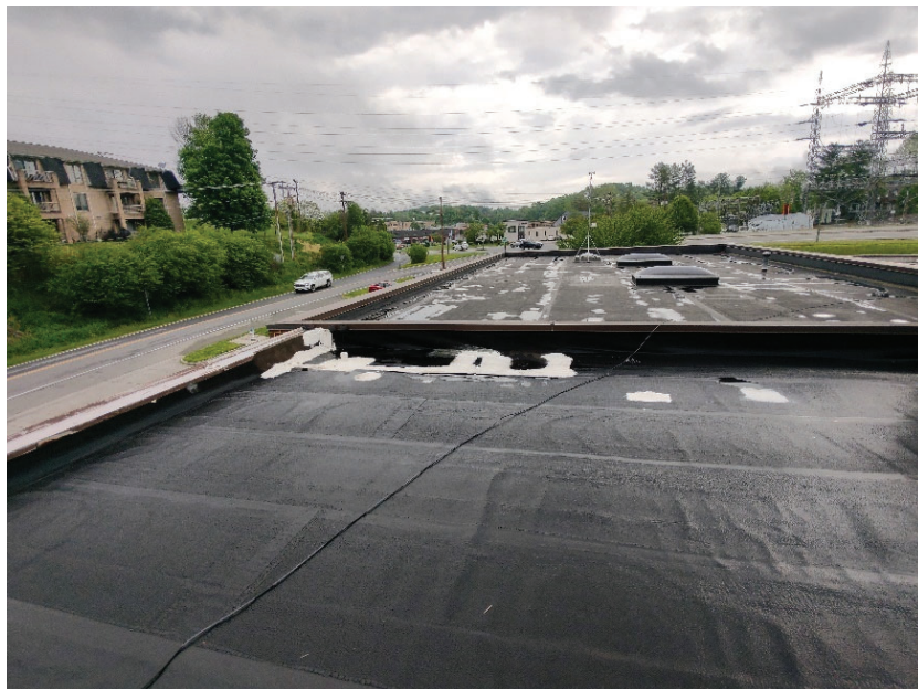
Figure 12, modified bitumen roof over insulation.
