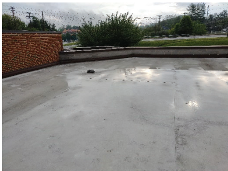
Figure 2, minimal roof slope
