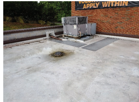
Figure 4, showing the rooftop unit with walkway pads surrounding the unit.
