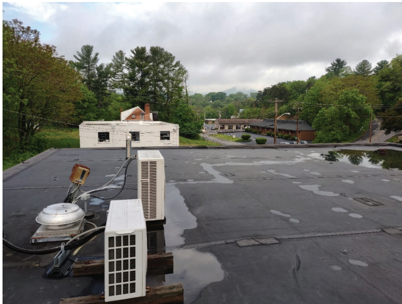
Figure 15, showing the fan coil rooftop units in the middle along the plan north side of Roof Five. Showing the other drain on the plan south side of the roof.
