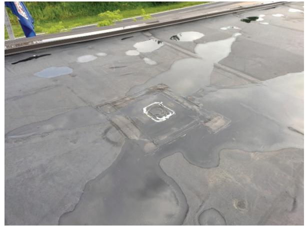
Figure 14, showing where there is a patch over where the drain in the middle of the plan south side used to be.
