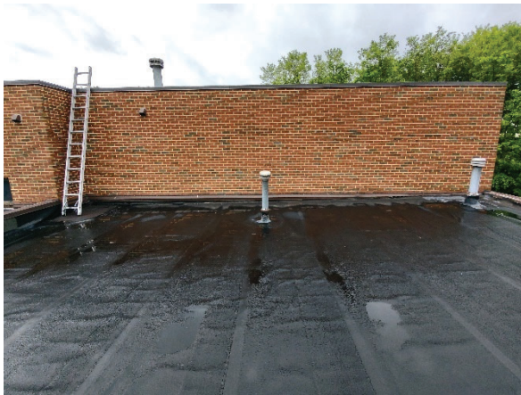
Figure 10, showing the modified bitumen roof over insulation sloping from plan east to plan west.
