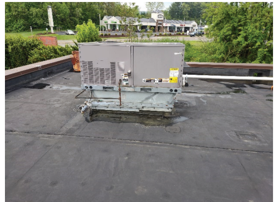
Figure 21, showing the roof top unit having no walkway pads.
