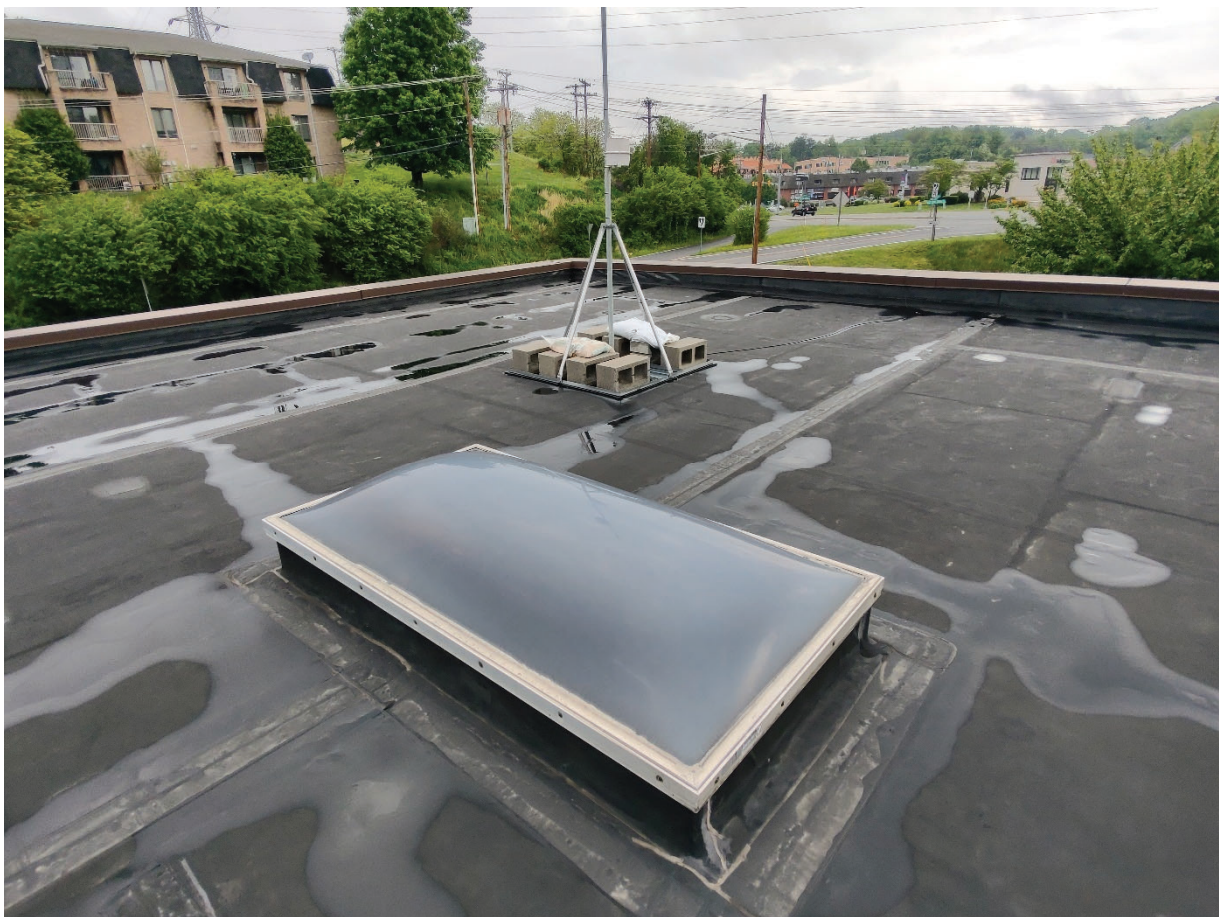
Figure 9, the roof showing ethylene propylene diene monomer (EPDM) on insulation, and one of two skylights on roof, with a weather station on roof weighed down with Concrete Masonry Units (CMU).
