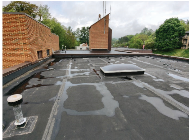
Figure 8, the roof showing ethylene propylene diene monomer (EPDM) on insulation, and one of two skylights on roof.
