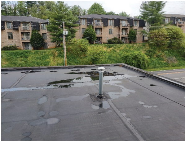
Figure 13, drainage along the plan south side of Roof Five.
