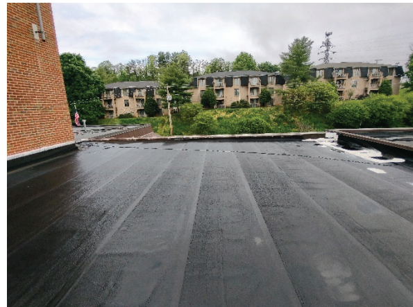
Figure 11, showing the roof patch work in the corner of the joining wall of Roofs Three and Four.
