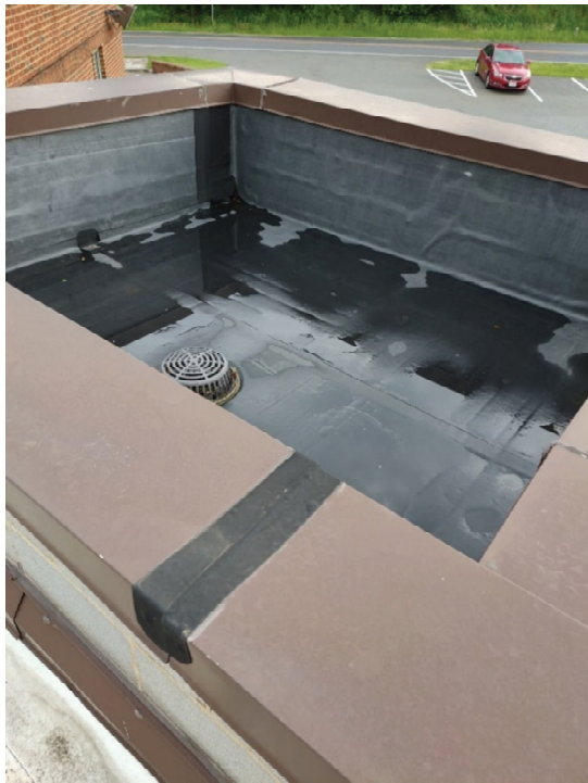
Figure 5, the roof showing ethylene propylene diene monomer (EPDM) on insulation and water flowing to roof drain.
