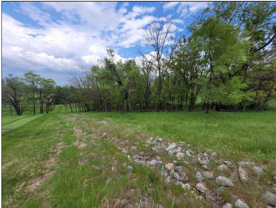
10 - Stormwater drainage ditch
