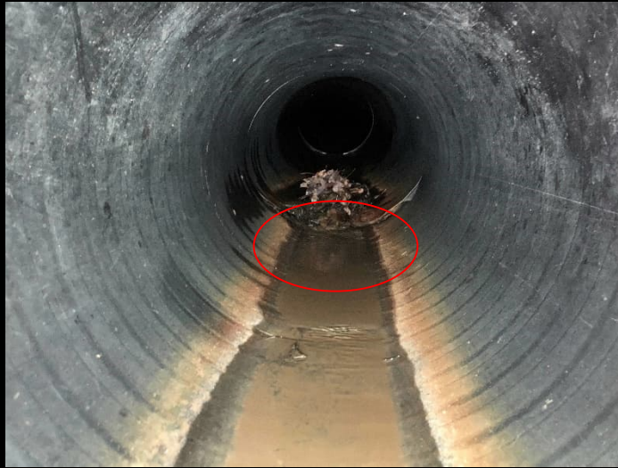
Photograph 21. Terminal End of Piping Diverting Stream Around Buried Fly Ash – Possible Crack at end of Plastic Corrugated Piping (Looking South).
