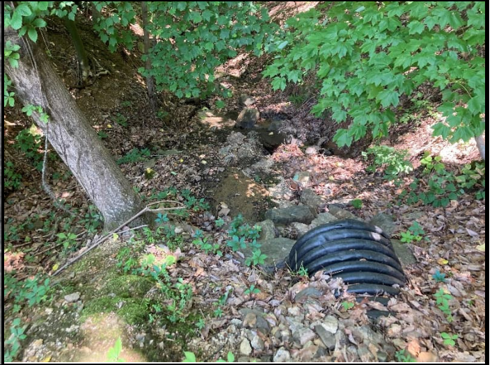
Photograph 22. Drainage from Piping Diverting Stream Around Buried Fly Ash (Looking South)
