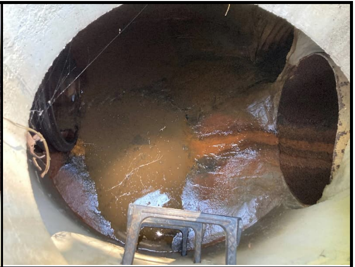
Photograph 20. Conveyance Lines Diverting Stream around Buried Fly Ash.
