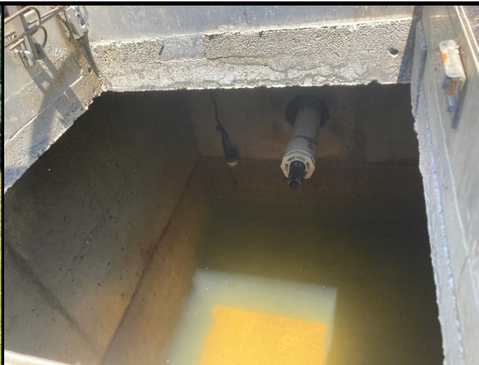
Photograph 26. Leak Detection Tank.
