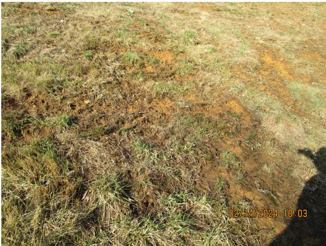
Downstream Face of Dam, Moist Seep Area
