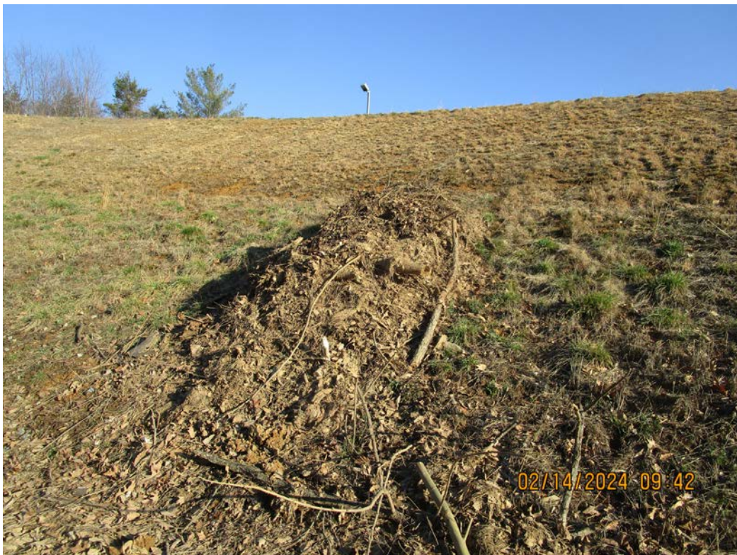
Minor debris on Upstream Dam Face
