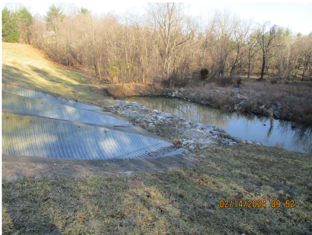
Plunge pool at emergency spillway outlet.
