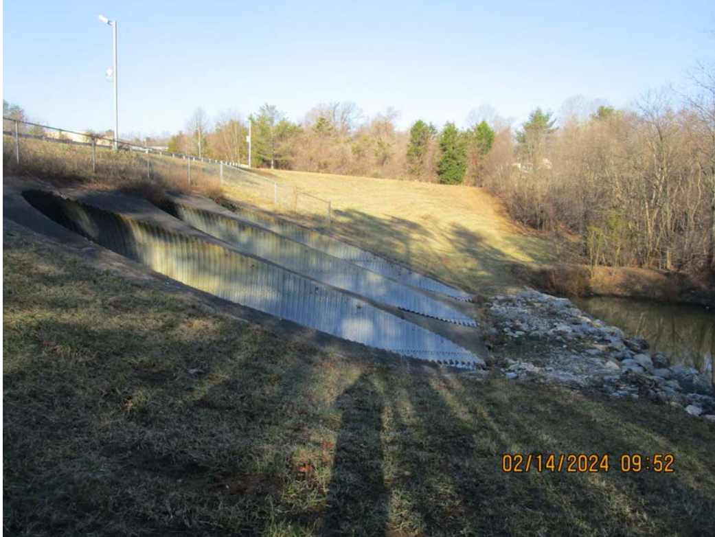
Downstream Face of Dam
