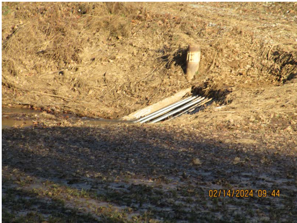
Intake structure. Note inlet is clear, with no debris.
