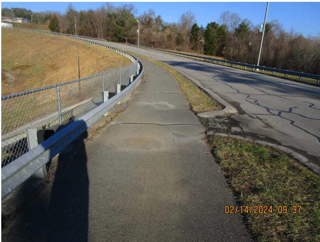
Looking overtop of Emergency Spillway Culverts, Note Settlement to Asphalt Trail
