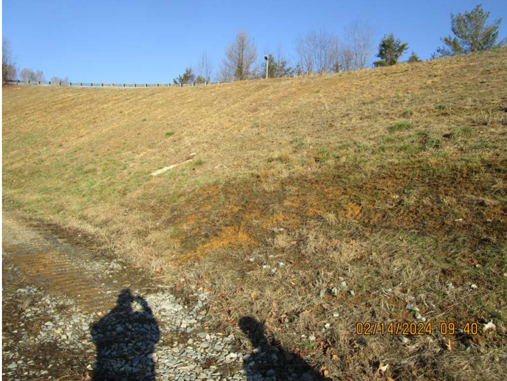
Looking at Upstream Dam Face, toward North Abutment- slight seep noted
