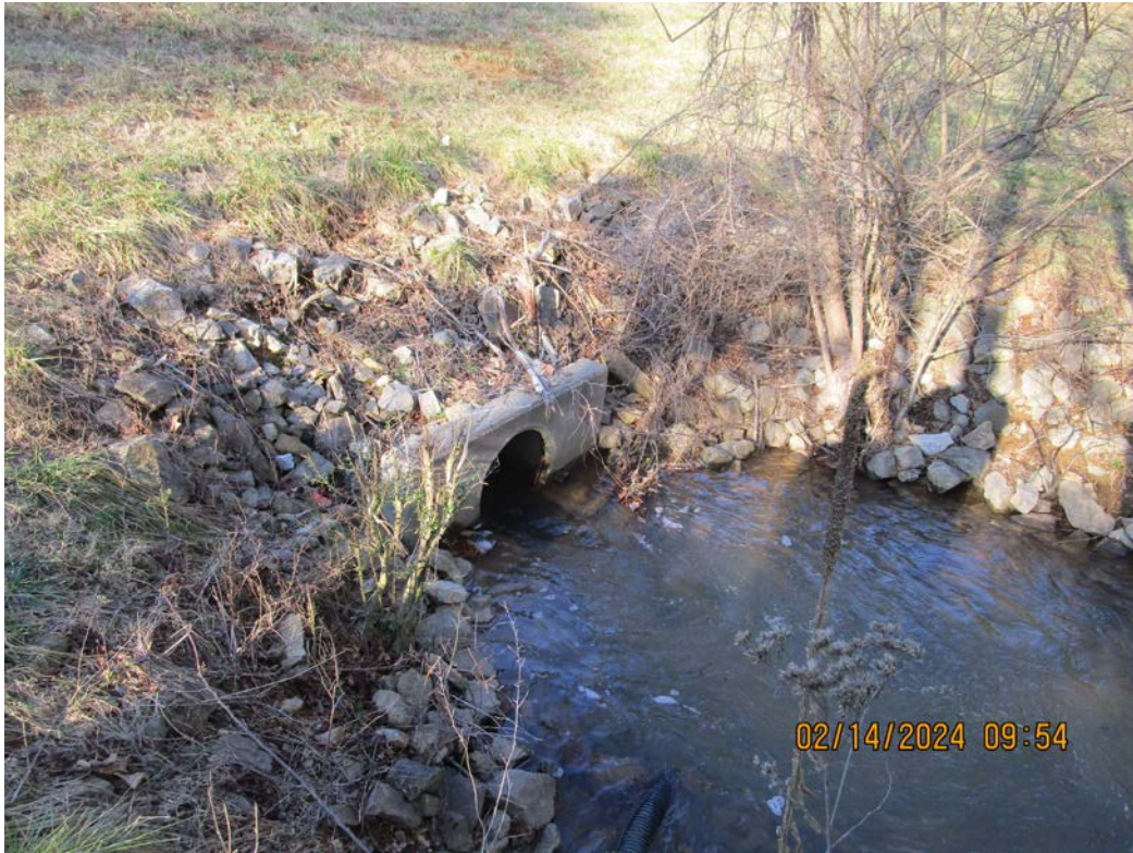
Looking Upstream at Discharge from Principal Spillway Pipe
