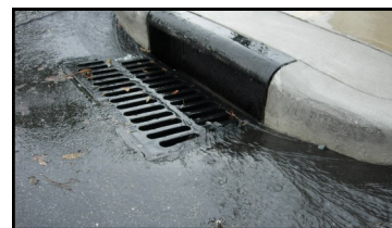
Pollutants reach streams thru storm drainage inlets and underground pipes.
