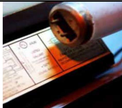
**Older Fluorescent light ballasts (FLBs)** can contain PCBs. Because of this, FLBs should be removed and disposed of by trained professionals.
