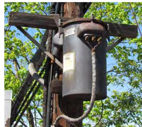
**Transformers containing PCBs**, which contain more than 50 ppm of PCBs, are subject to specific EPA regulations. Proper PCBs identification labels must be visible near the access and on the transformer itself.
