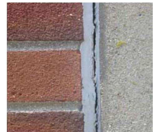
**Old paint and caulk** and surrounding substrate (brick, masonry, cinder block, wood, etc.) contain PCBs. Care must be taken during removal of these materials to avoid the creation of dust and to contain contaminated waste.
