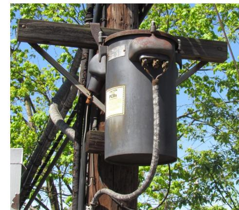
**Transformers containing PCBs**, which contain more than 50 ppm of PCBs, are subject to specific EPA regulations. Proper PCBs identification labels must be visible near the access and on the transformer itself.
